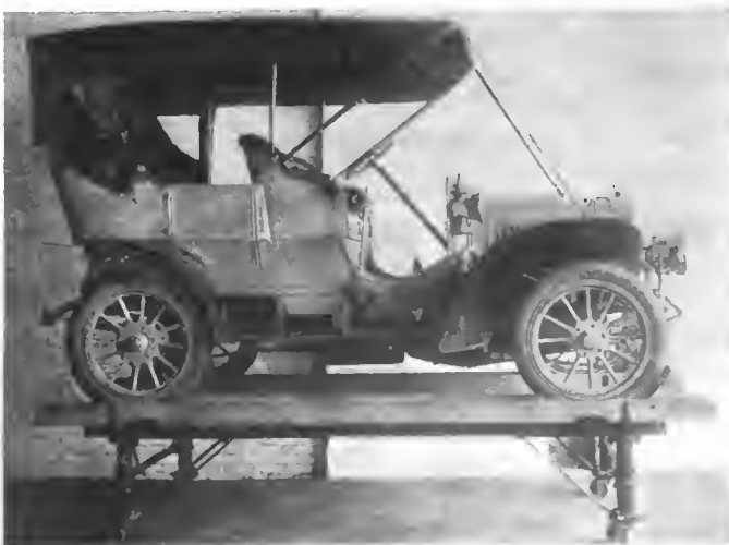
HANDY TRUCK DESIGNED TO REPLACE PITS IN GARAGES.
